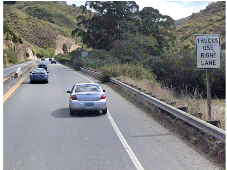
Google Street View of Highway 92
