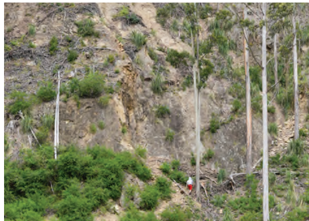
Quarry wall erosion
