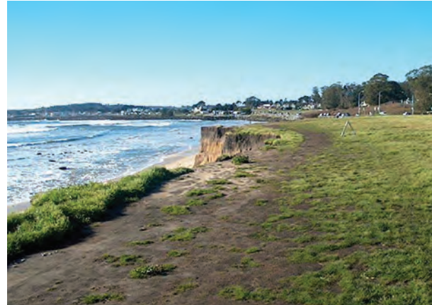
Bluff erosion at Mirada Surf West (Coast)
