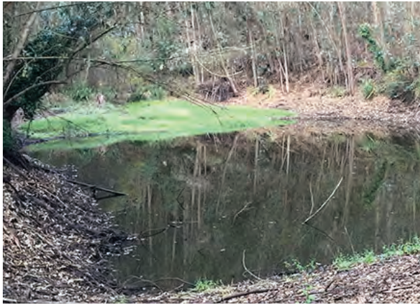
Reservoir and Earthen Dam
