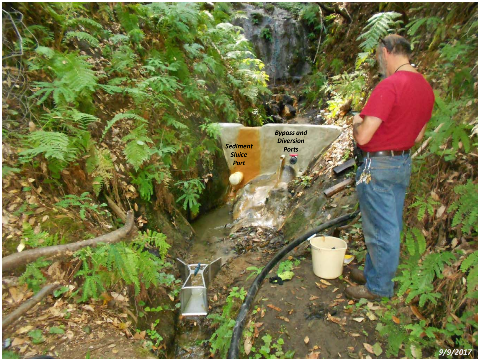
Figure 2. Diversion structure on Piney Creek, Redwood Glen, San Mateo County, CA. The diversion structure consists of a concrete dam across a narrow (4-ft.) bedrock notch, which includes a 2-inch diameter diversion port and bypass port, and a 4-inch diameter sediment sluice port. Twice annually the sluice port is opened and sediment is flushed downstream.
