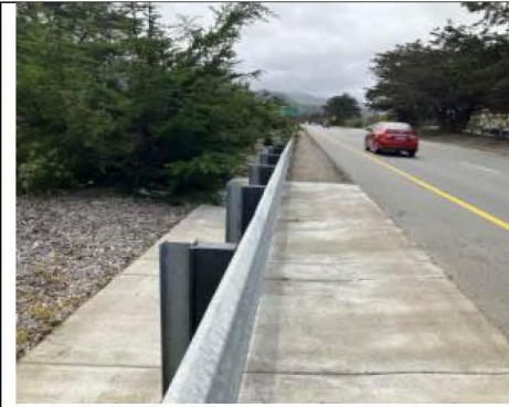
Photo 1: Pacifica Midwest Guardrail System on SR-1 with concrete surround.
