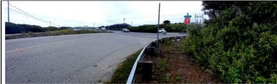
Photo 5: Existing guardrail at Capistrano Rd. (north) composed of metal and treated wood adjacent a riparian corridor. This guardrail serves no purpose and was installed prior to the addition of a southbound off-ramp roadway built for vehicles to safely round the corner at higher speeds as they enter into the Harbor.
