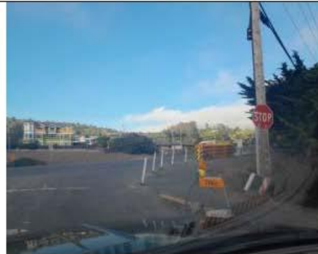
Photo 7: SR-1 at Medio needs sufficient work to upgrade current conditions. Describe this work and materials proposed in detail.
