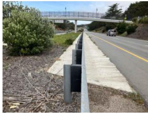
Photo 2: Pacifica Midwest Guardrail System on SR-1 with concrete surround.
