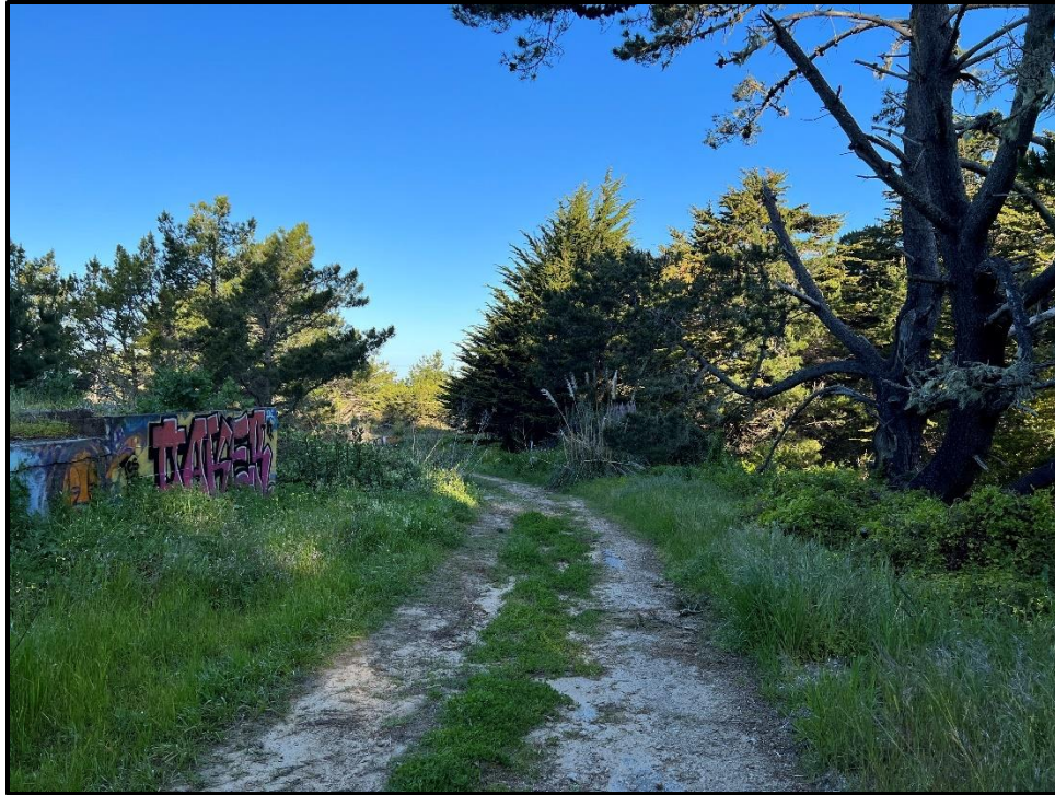
Photo G-3. View facing northwest showing a dirt access road, adjacent concrete foundation (left), and perennial rye grass and Monterey cypress – Monterey pine vegetation communities in the northern portion of the BSA. Photo taken April 4, 2023.
