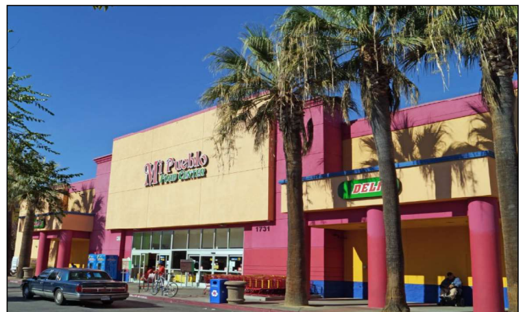
Mi Pueblo Food Center - Ravenswood 101 Shopping Center Photo courtesy of County of San Mateo
