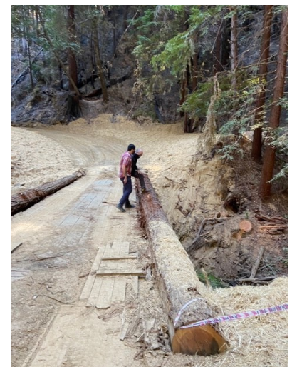
Trestle Creek Bridge Reinforcement © County of San Mateo
